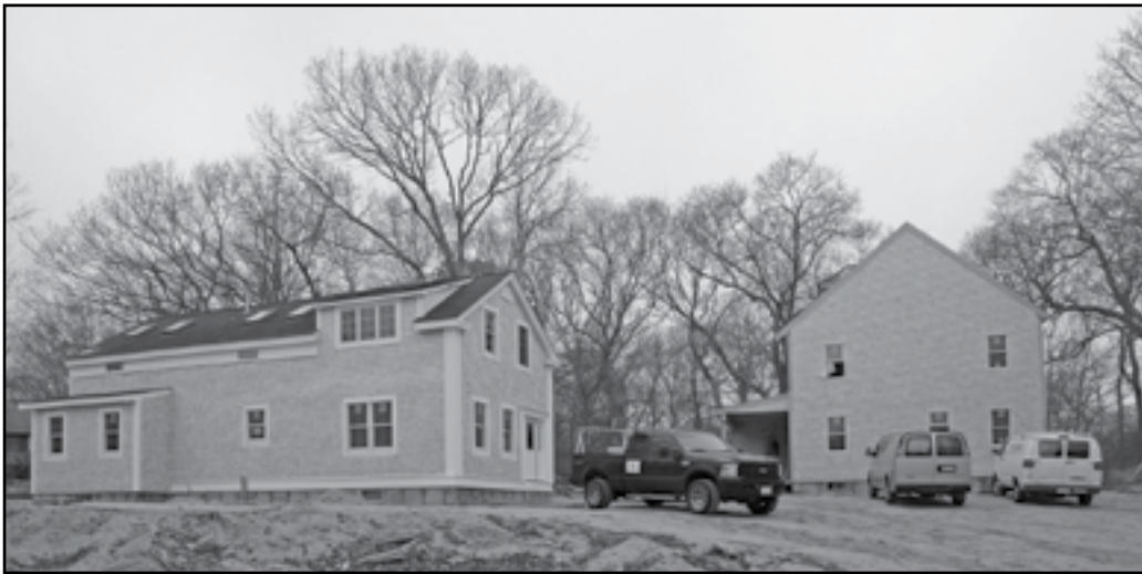
New homes nearing completion at 150 State Road in Vineyard Haven.
